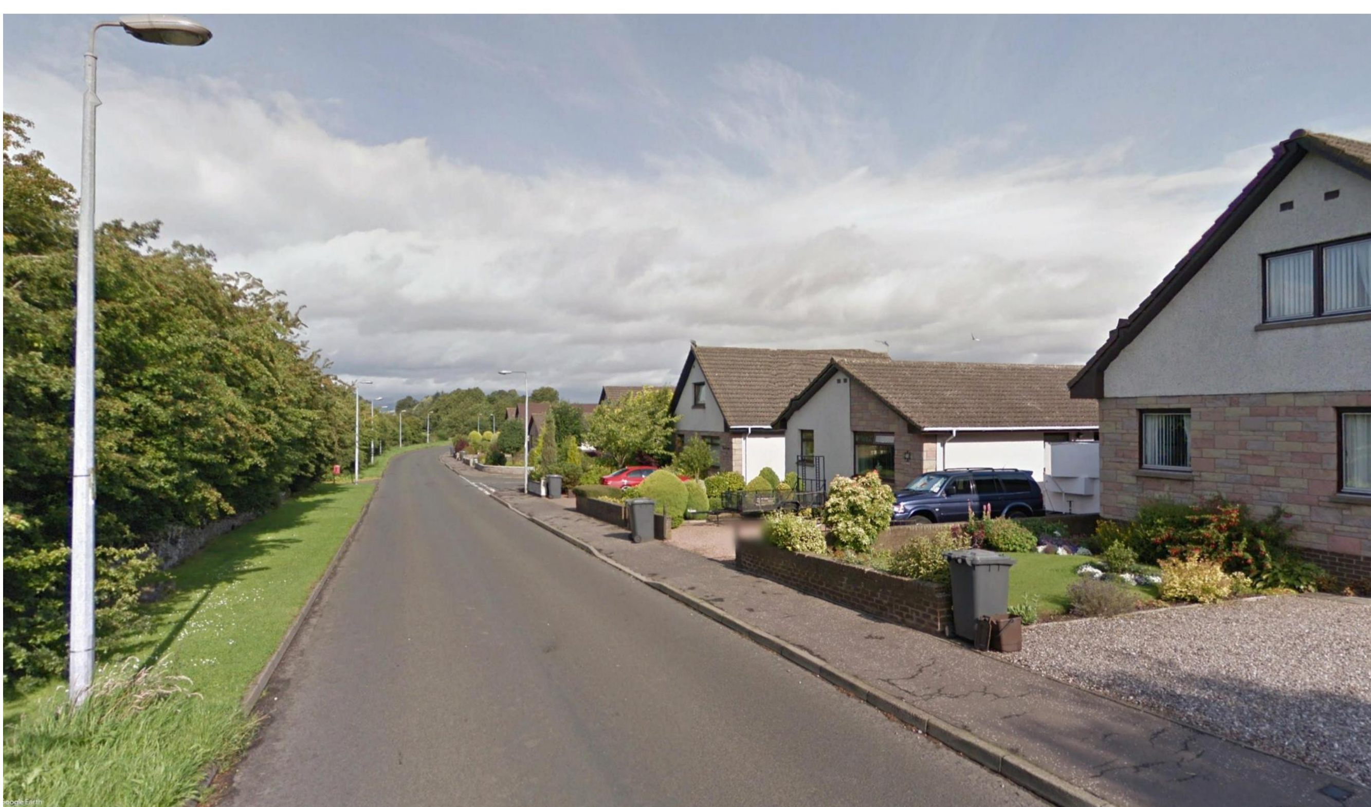
Existing housing along Westfield Loan
