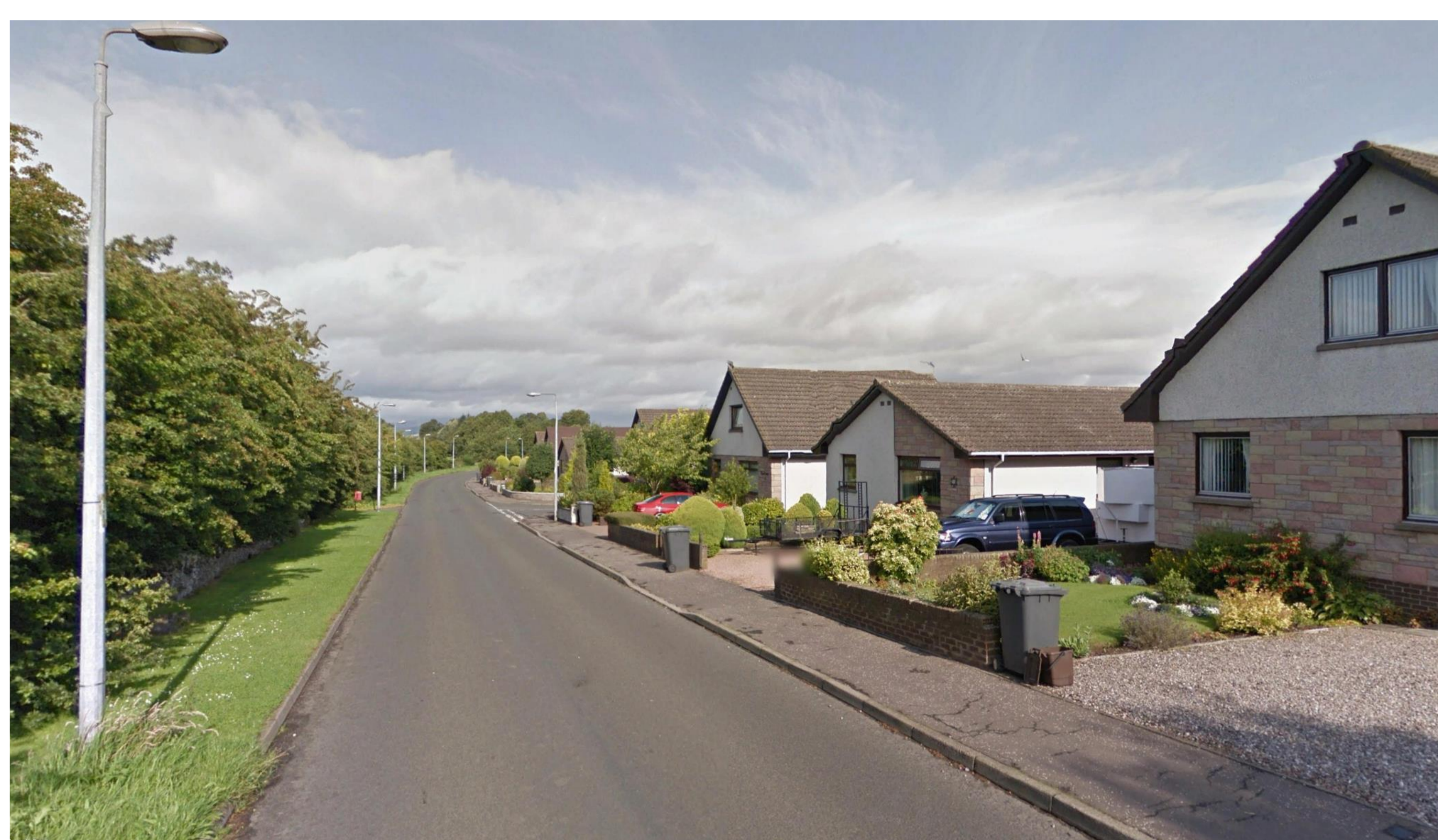
Existing housing along Westfield Loan
